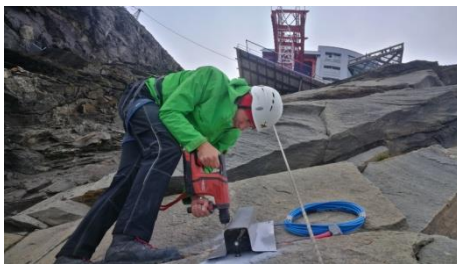
Drilling a hole for the extensometer
